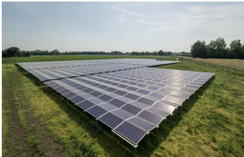
Figure 2. The PEG mounting structure comprises rows of alternate facing modules (photo courtesy of Belectric, n.d.)
